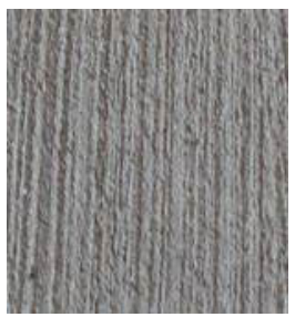
Unsealed Brushed Concrete
